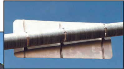
Mast Arm Sign Installation
