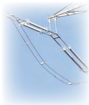
420 kV Suspended Double Tension Set
