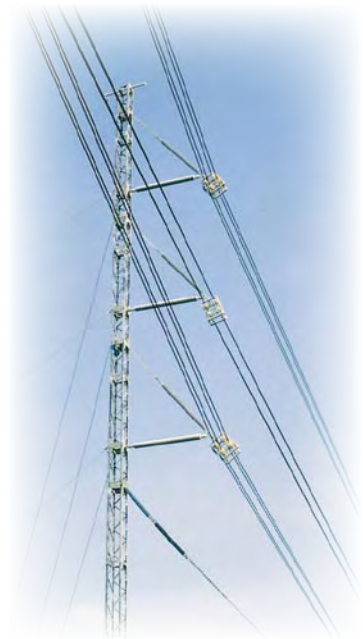
Insulated Crossarm for 420 kV Emergency Tower
