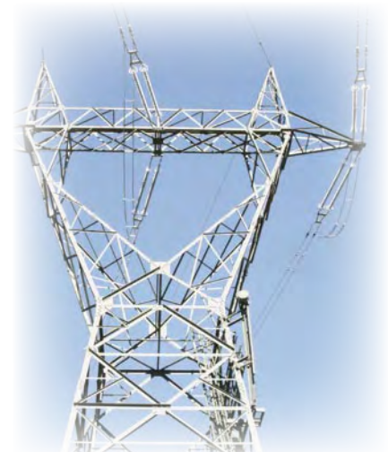
ATEL's 420 kV Line with 500 kN Force Rating
