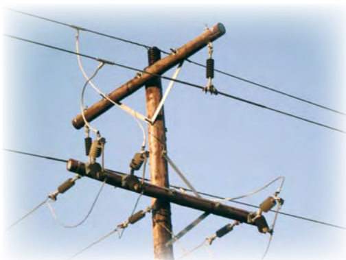
Wood Pole with Suspension and Tension Insulators and Cutouts
