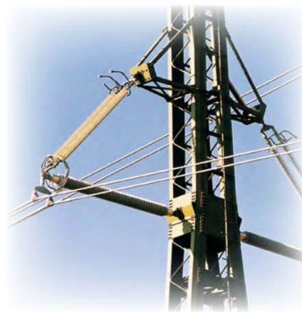
420 kV Braced Line Post erected in 1998
