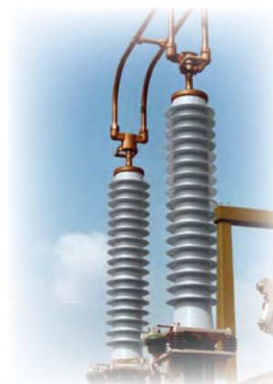
123 kV Cable Termination installed in 1975
