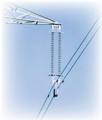
420 kV Double Suspension Set
