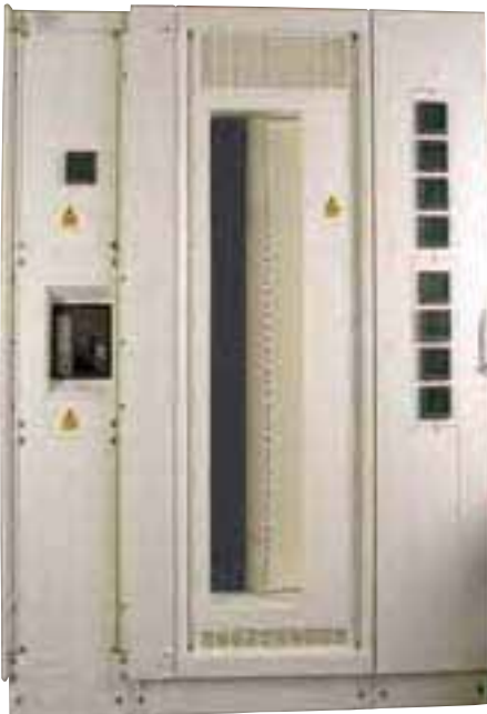
1600A panelboard with metering on side extension
