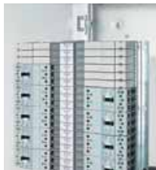
Totally enclosed busbar system rated at 400A
