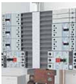
Totally enclosed busbar system rated at 800A
