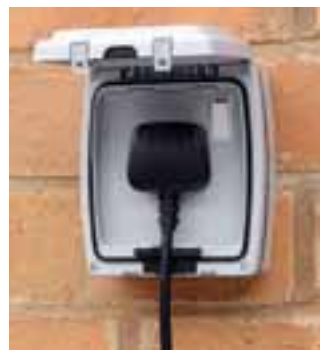
The neoprene seals will not stain the cable.
