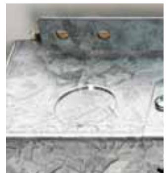
Back box can be fitted either way to allow choice between 25 or 32mm knockout for incoming.
