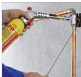
Hard soldering in refrigeration and climate control
