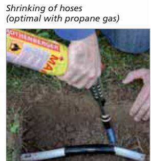
Shrinking of hoses (optimal with propane gas)
