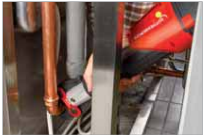
Work in confined spaces
