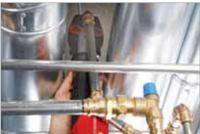
Work over head
