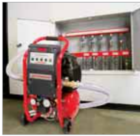
Cleaning of floor heating
