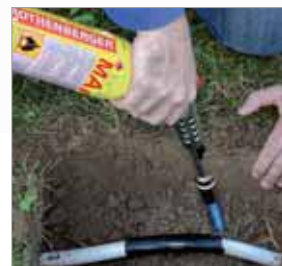
Shrinking of hoses (optimal with propane gas)
