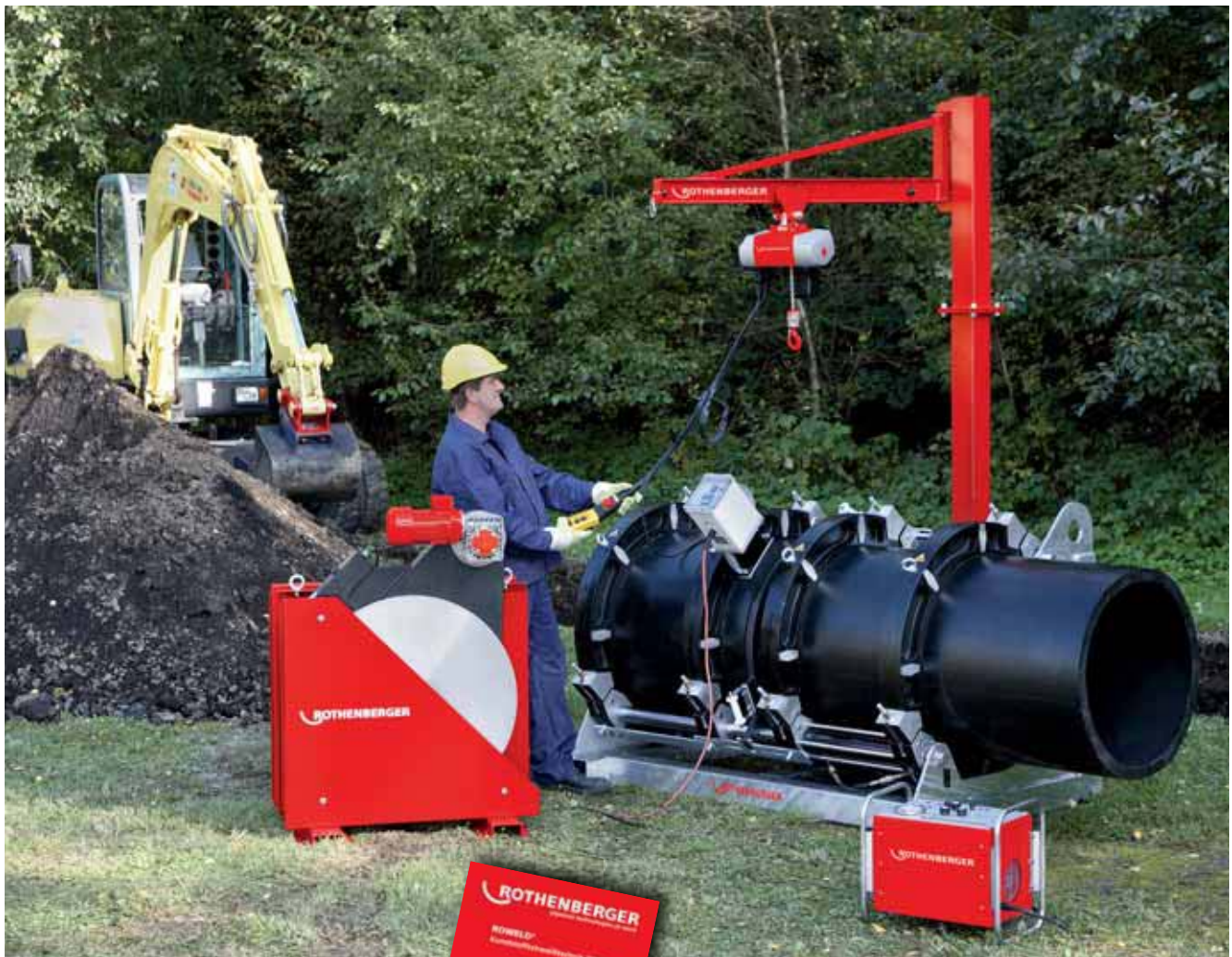
ROWELD® P 800 B with electronic life-out device
