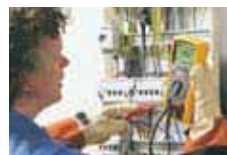
Insulation test at a distribution panel
