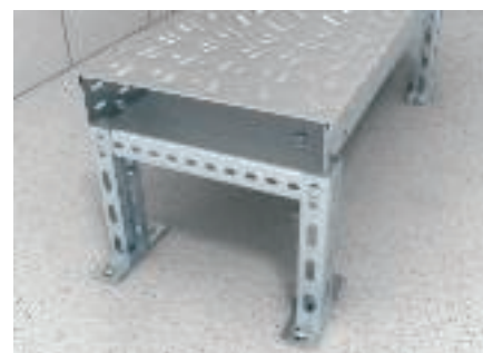
Installation and fastening of the walkable cable tray system for floor stand-off.
